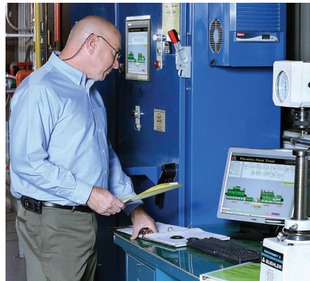
Peter Hushek verifies automated processing control set points before heat treating a fastener job. The programmable logic controllers automatically run every system in the continuous cast link furnace.
